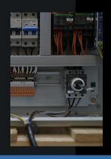
POWER: The same Telemetrix panel can take either 230V or 400V (with no neutral required).
